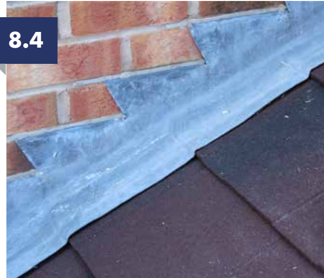
Reposition the existing lead to complete the external installation
